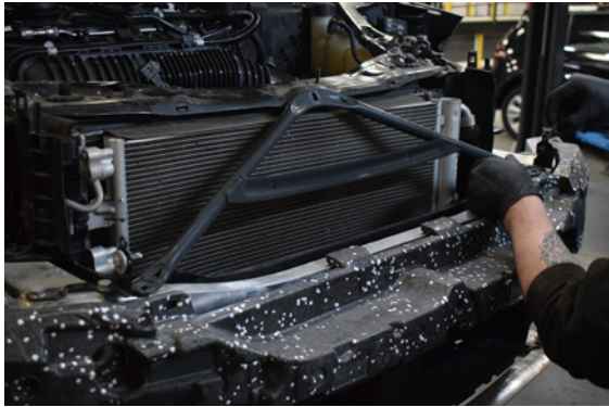
99. Install front brace.
