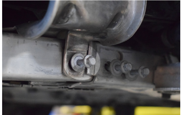
76. Install final bolt to secure the side bracket.
