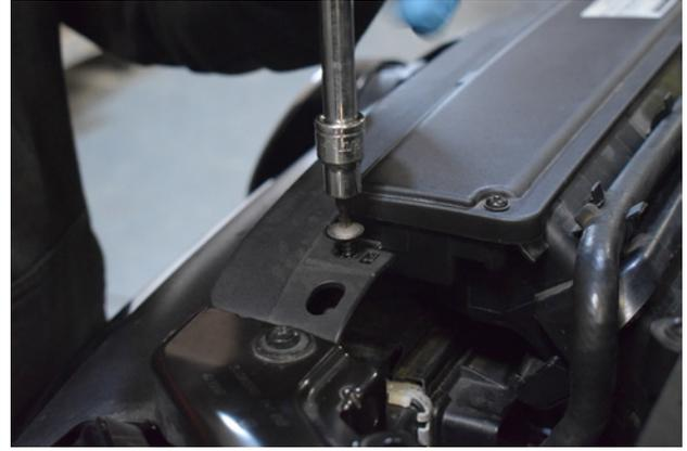
2. Undo the 2x upper screws on the plastic trim panel.
