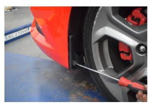
52. Re install 4x screws under inner wheel arch.
